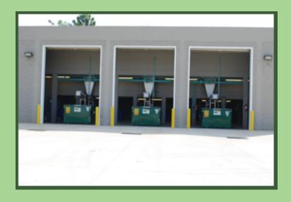
1 Headwork Building - this building houses three internally fed drum screens with dewatering press augers. This system is used for the removal and dewatering of grit and screenings. Each screen has a capacity to process twelve million gallons per day. The dewatered material from the screen is emptied into dumpsters and taken to the landfill for disposal.
