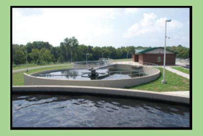
**3** Clarifiers - these structures allow solids present in the discharge from the Oxidation Ditches to settle and be removed. A clear effluent from the clarifiers flows over the weirs and onto the Polishing Clarifiers. The settled sludge is either pumped back into the Oxidation Ditches or to the Digesters for further processing. There are four clarifiers at the Gallatin Wastewater Treatment Plant with a combined volume of approximately 3.75 million gallons.
